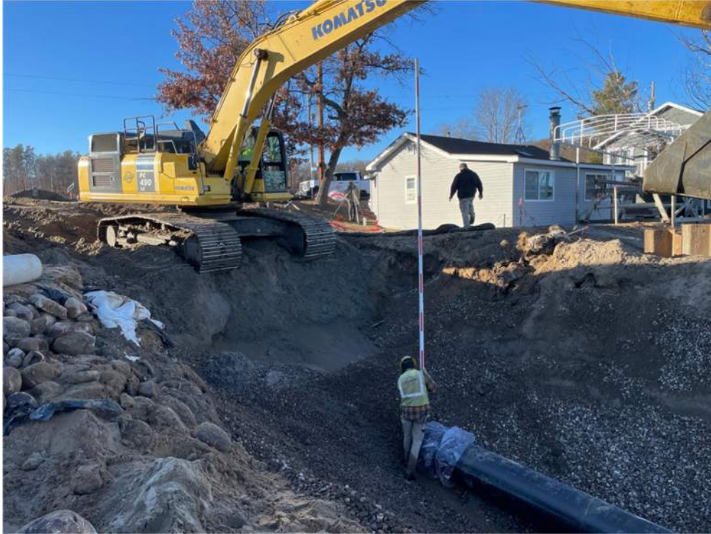
Photo #7: Verifying elevation of pipe - Dec 7, 2023, 2:39 PM
