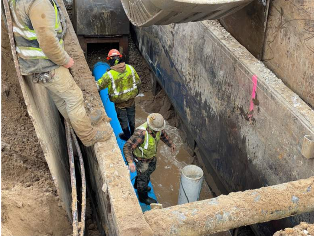
Photo #3: Force main pipe installed - Dec 5, 2023, 10:55 AM
