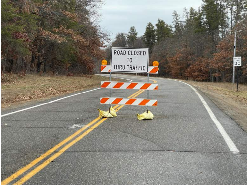
Photo #9: Traffic control signs back in place for closure of Aztec Road - Dec 8, 2023, 1:38 PM
